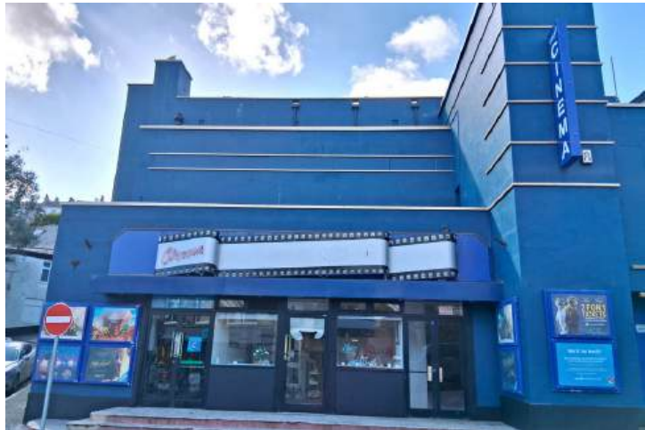
The Royal Cinema has re-opened in St Ives after a major refurbishment, involving new seating and updated toilets and air conditioning. Work was part-funded via a St Ives Town Deal grant.
