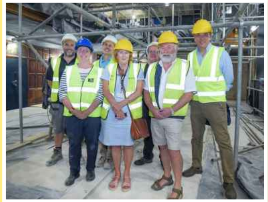
Representatives of Cornwall Council and the St Ives Town Deal Board are shown work in progress at the theatre by architect Clare Mackness.
